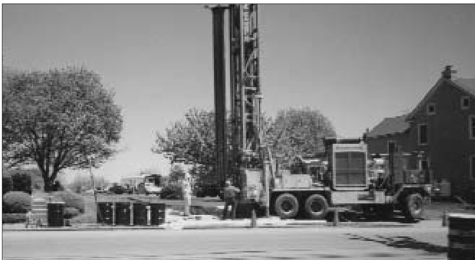
Off-site recovery well installation
