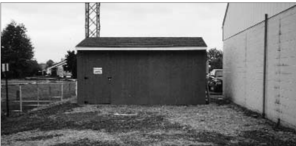
Remediation system upgrade
